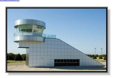
Construction Method: Steel w/ ReynoBond Panel System Cladding –Structural Steel Cab
