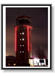
Construction Method: Structural Precast Concrete Shaft; Steel Frame Cab
